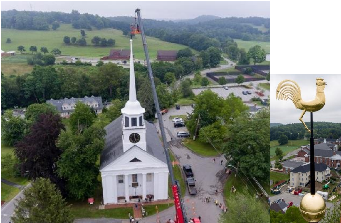
Figure 8: First Parish Restoration – Buddy Installation
